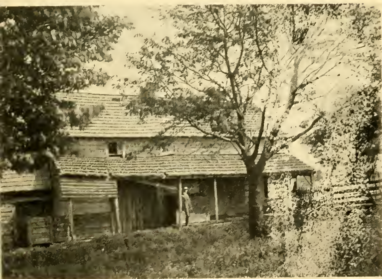
OLD FORT GADDIS, NEAR UNIONTOWN, PENNSYLVANIA
